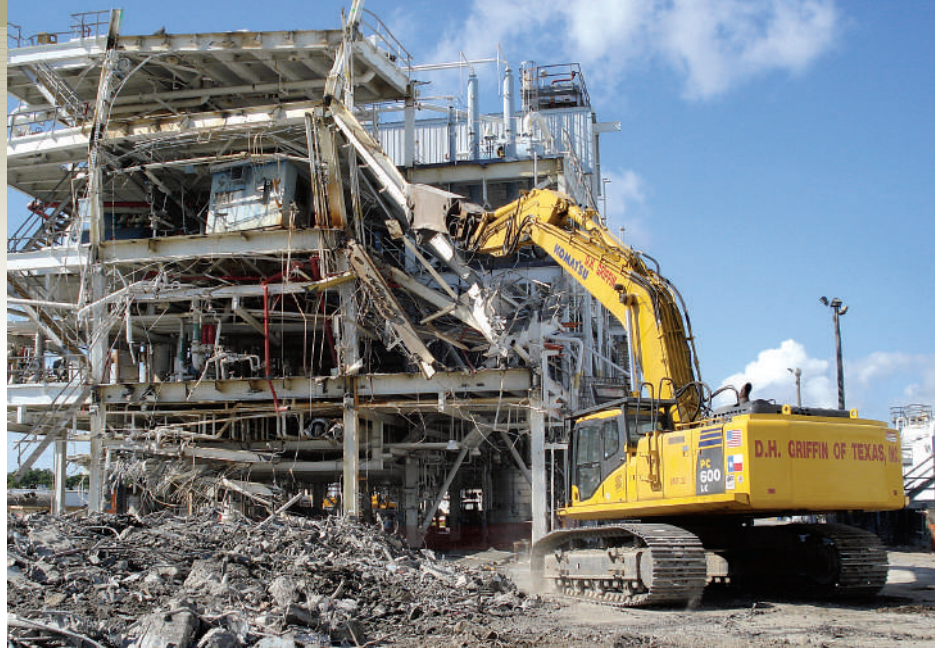
Using a new Komatsu PC600LC-8 excavator, equipped with LaBounty shears, a D.H. Griffin of Texas operator demolishes a building. "We use the excavators in every facet, including digging the pits for implosions, loading trucks, processing scrap materials with the shears and hammering," said President John Angelina.
